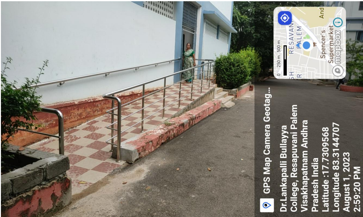
Ramp ways for Divyangjan
