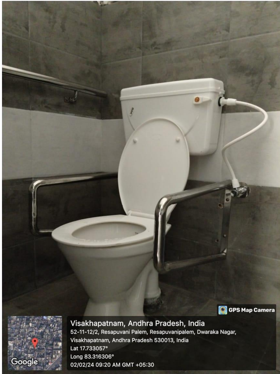
Toilets for Divyangjan
